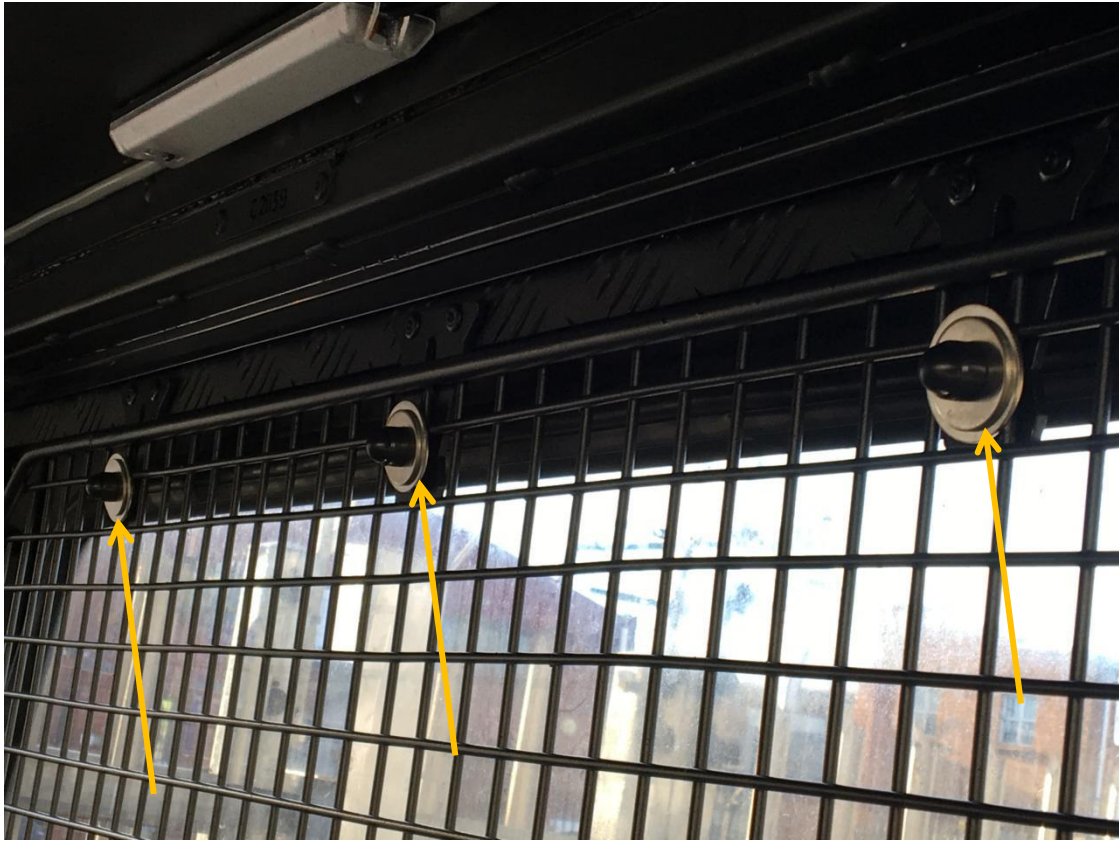
Figure 10: Spaced out Top Vertical Mounts installed
